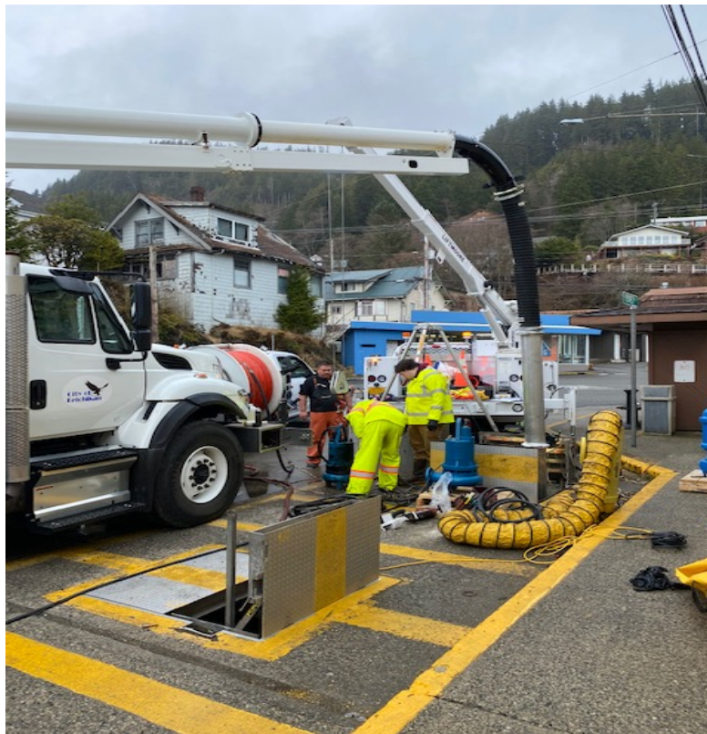
Wastewater Collection Crew Swapping a Submersible Pump at Station 3
