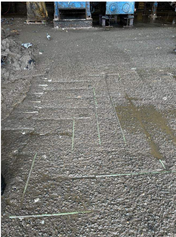
Solid Waste Tipping Floor – Exposed Rebar
