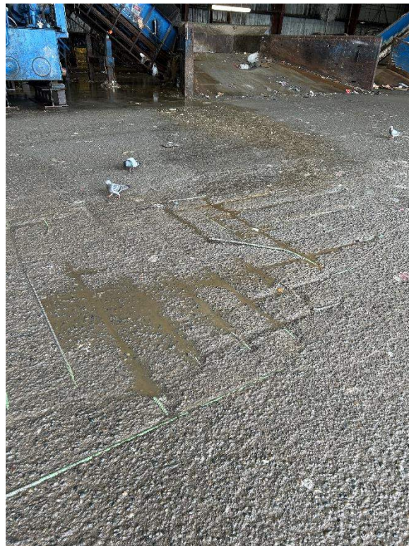
Solid Waste Tipping Floor – Exposed Rebar
